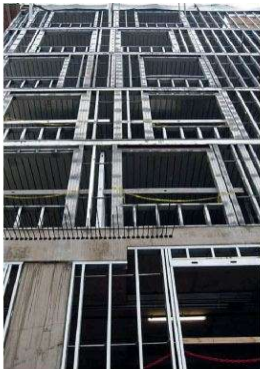
Fig.1.3 Mid-rise CFS framing
